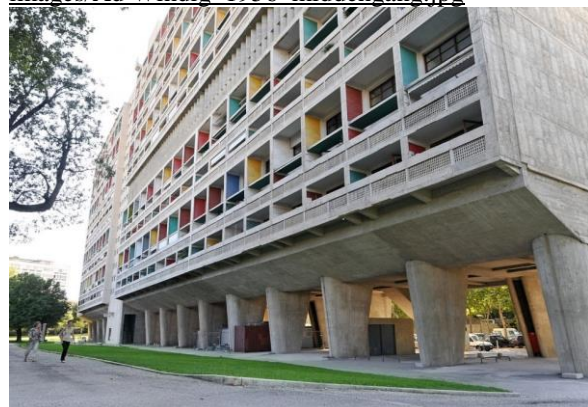
Afb. 3.7 Detail betonnen kolommen begane grond Unité d'Habitation. Foto: Shelley Davies http://shelleysdavies.com/unite-dhabitation/
